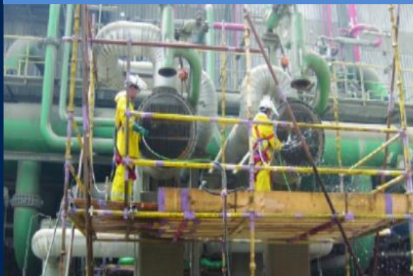
Shutdown Maintenance of Heat Exchangers - EFC
