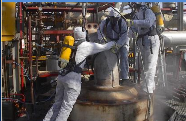
Maintenance of Hydrocracker Reactor
