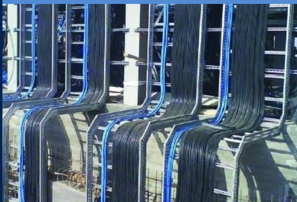
Installation of Instrument Cables
