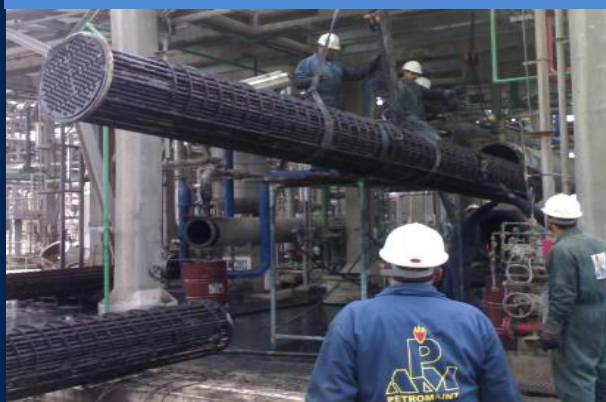
Maint. of Heat Exchangers
