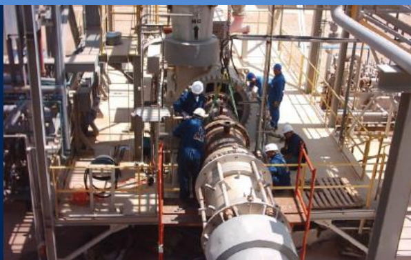
Shutdown Maintenance of Compressor - OPC
